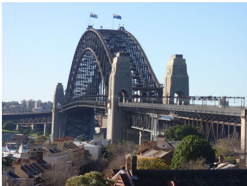
SYDNEY HARBOUR BRIDGE
